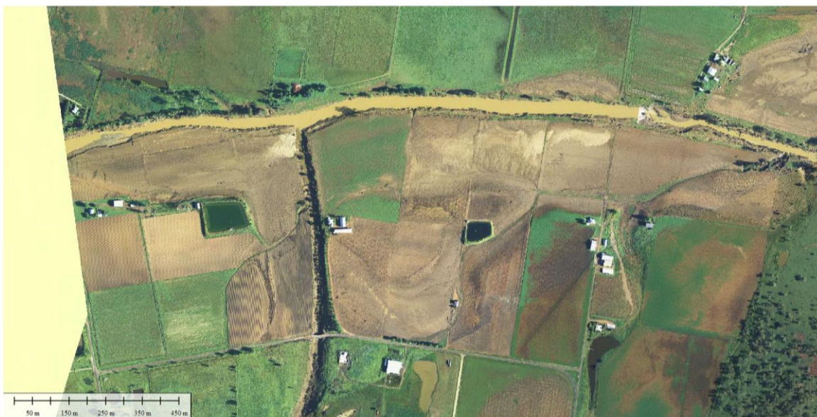
Figure 6.4 – Aerial Image of [REDACTED], Post Flood January 2011
